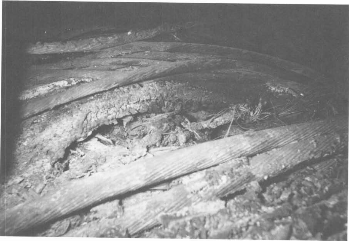
Photograph 3-10. Close-up of "pocket burn," Section 1.
