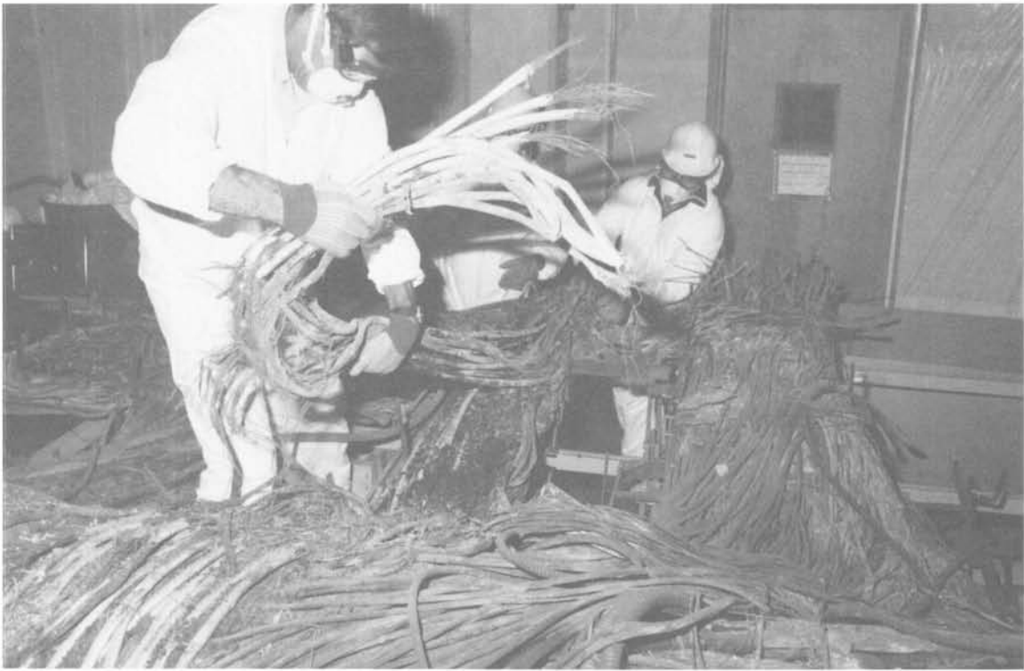
Photograph 3-11. Removal of communications cables from Section 1.
