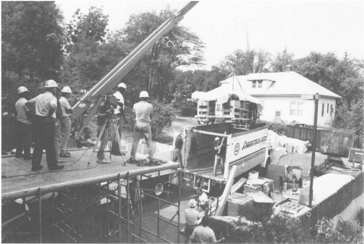
Photograph 3-43. Loading Section 2 into truck for transfer to storage facility.
