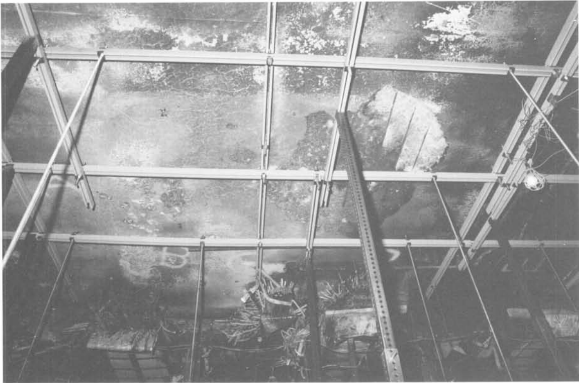
Photograph 3-4. Part of ceiling area above Section 1.
